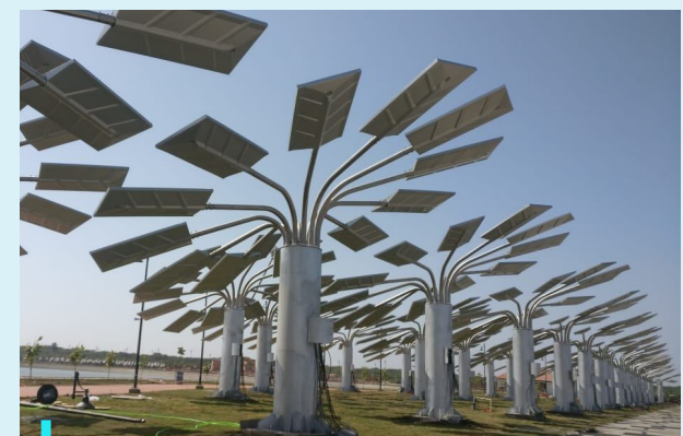
Energy for the entire memorial is generated from 41 solar trees developed by IIT Bombay and installed at the site. The energy generated would be fed into the grid during the day and the Memorial would then draw power from the grid at night, making it a Zero Energy initiative
